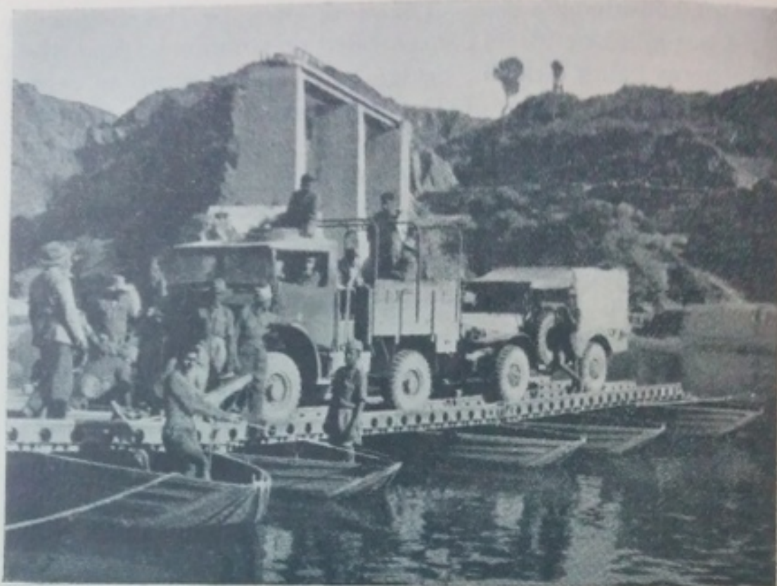
Ferrying trucks over a Bailey bridge at Beri Pattan.
